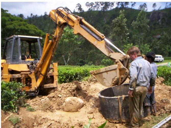
Digging and installing a water well, pump, pipeline and tank system for a local Primary school
